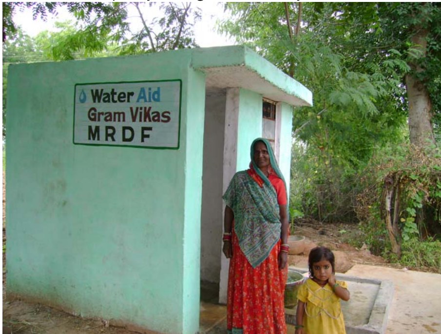
Picture 2: A woman proudly standing outside her newly constructed latrine, Suda, 2007
